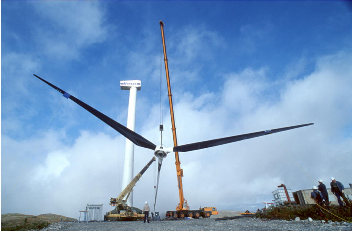
Photograph 9: the second wind turbine being installed
