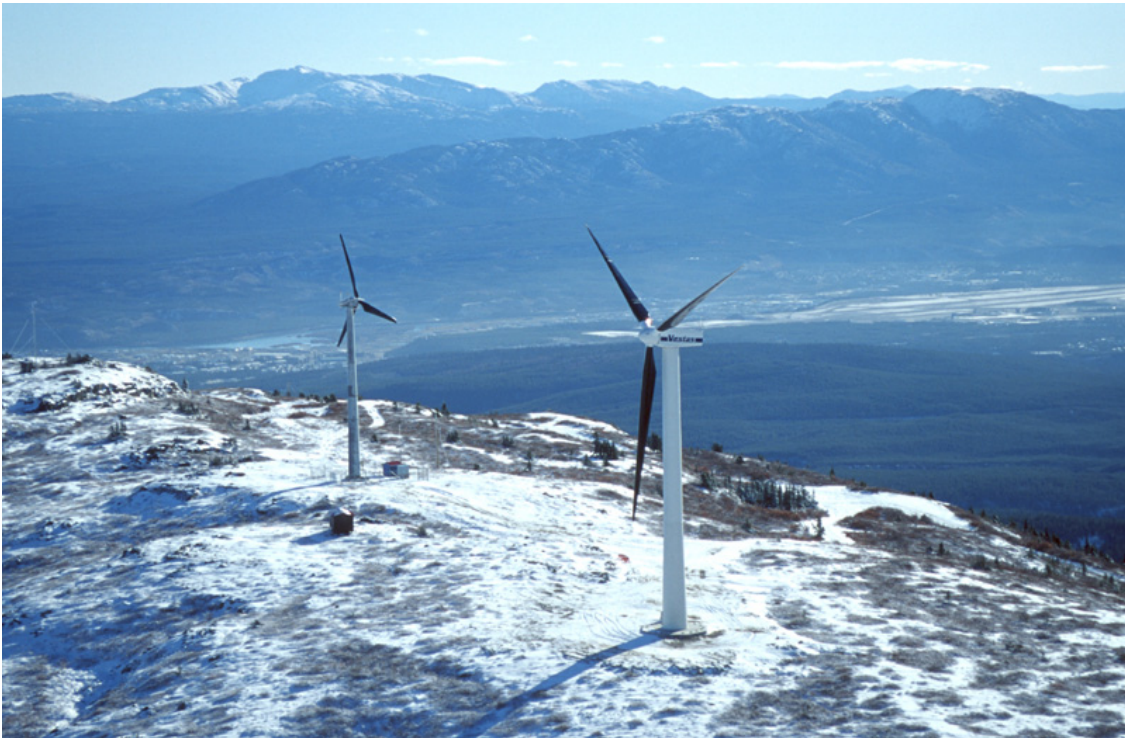
Photograph 10: both wind turbines in place
